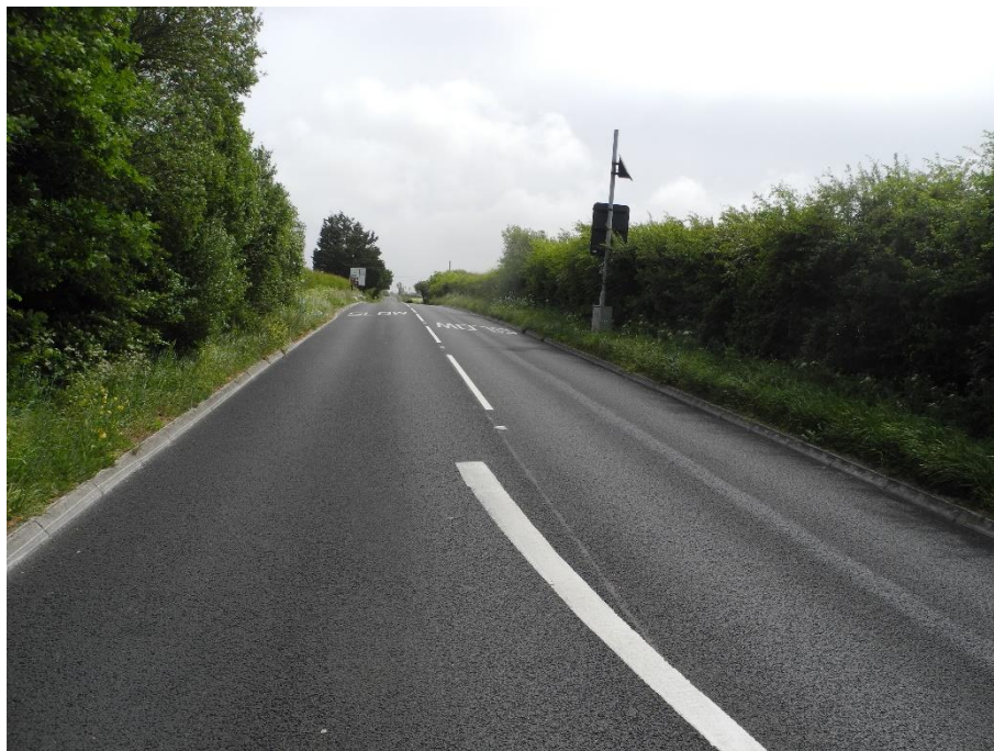
Image 5 – looking east approximately 160m west of junction
