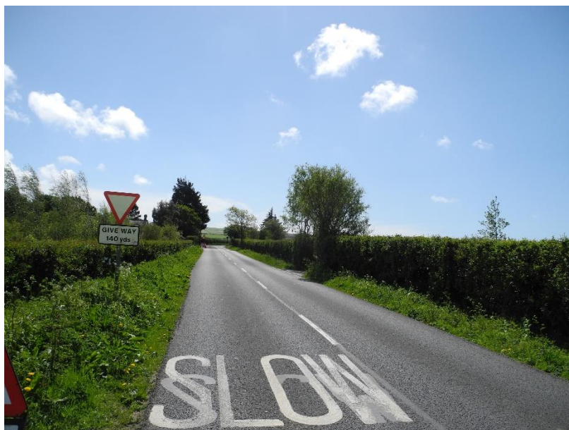
Image 2 – Advance give way sign and slow marking on Whitehouse Road approach
